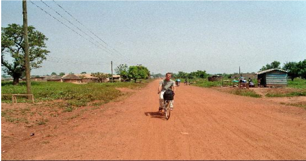
Figure 1.4: Picture of a Feeder Road
